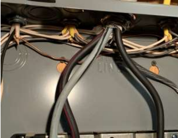
Figure 99 Improper connection
