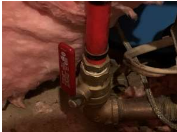
Figure 88 Main Water Shutoff
