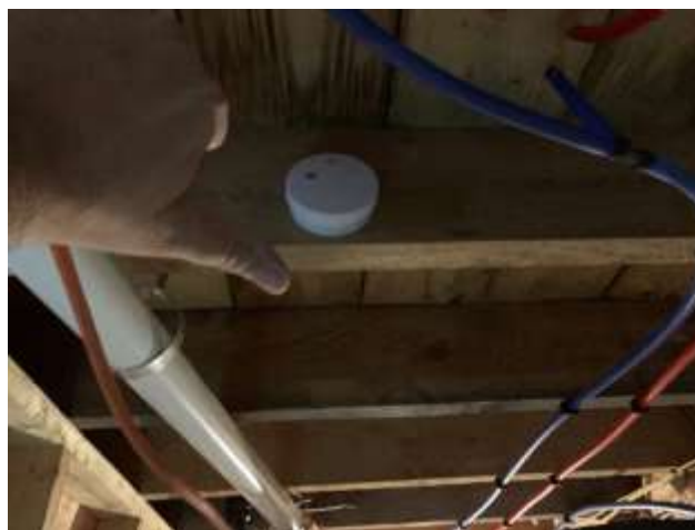
Figure 73 Inoperable Smoke Alarm
