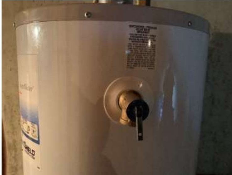
Figure 91 TPR Valve w/o termination
