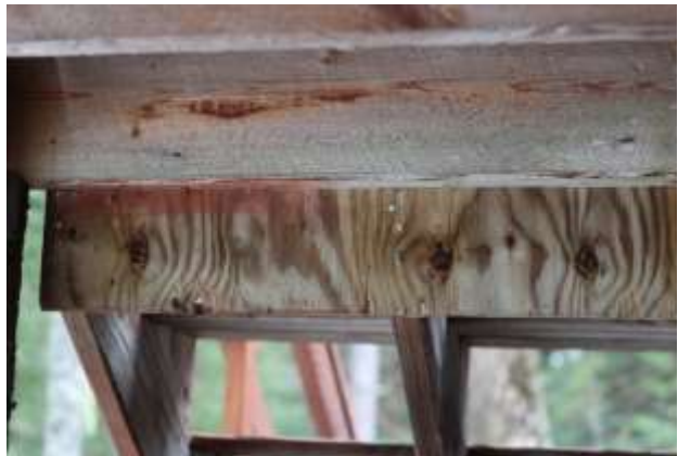
Figure 19 Improper attachment
