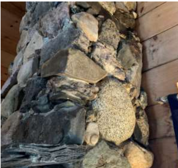
Figure 34 Water Staining
