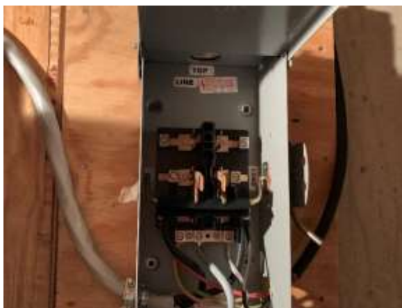
Figure 96 Generator Disconnect
