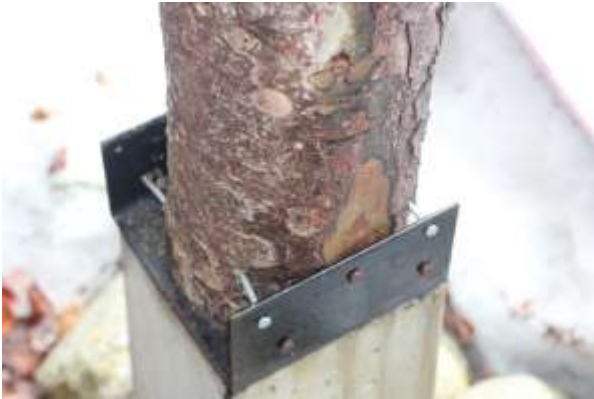
Figure 16 Improper materials
