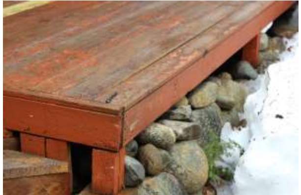
Figure 17 Lack of railing
