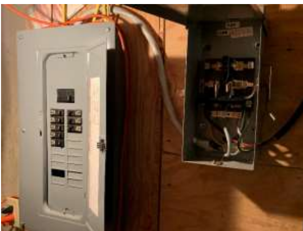
Figure 95 Main panel with generator disconnect switch
