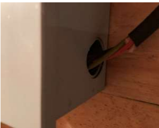
Figure 97 Improper fitting
