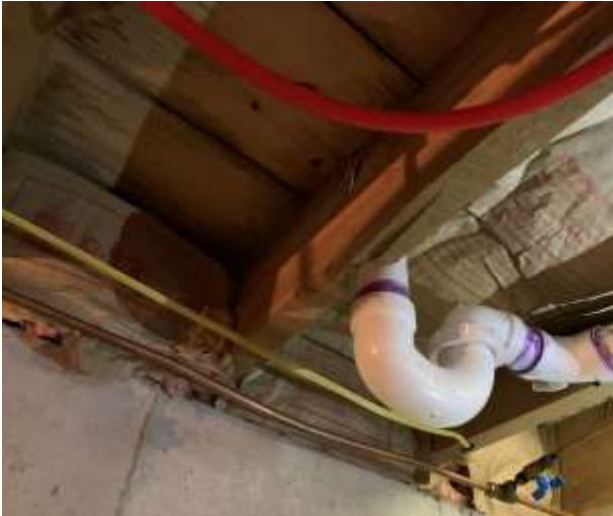
Figure 74 Cut Joist
