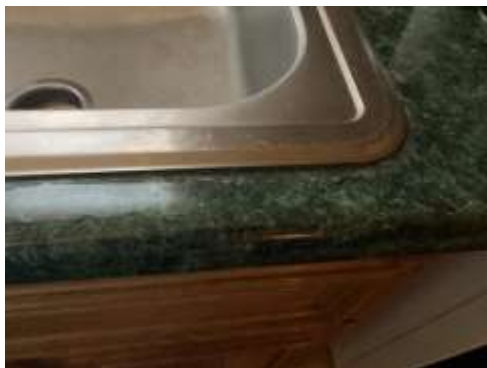
Figure 62 Loose Sink Connection
