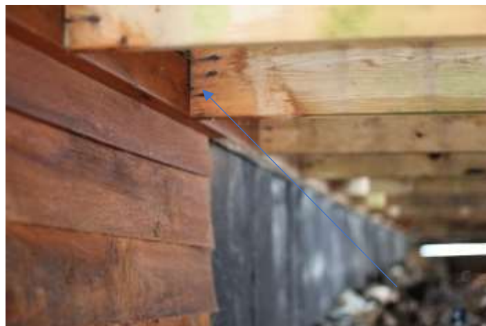
Figure 20 Lack of Joist Hangers
