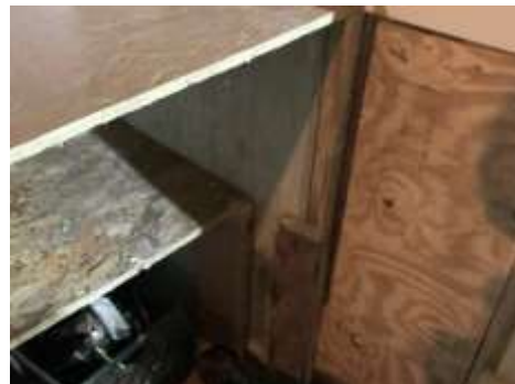
Figure 81 Active Water Intrusion
