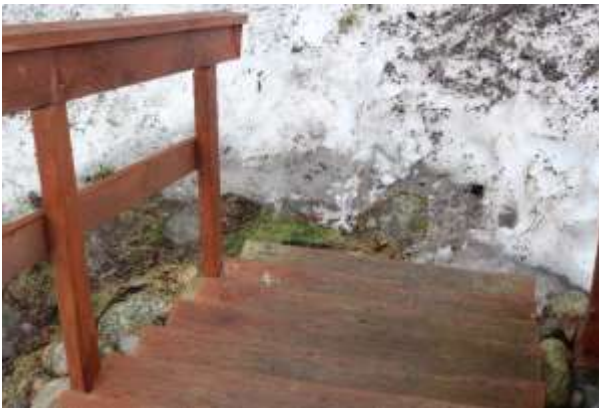
Figure 18 No Graspable Handrail
