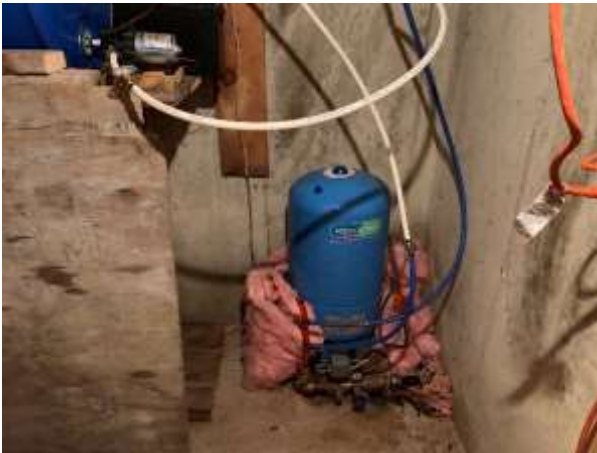
Figure 87 Pressure Tank
