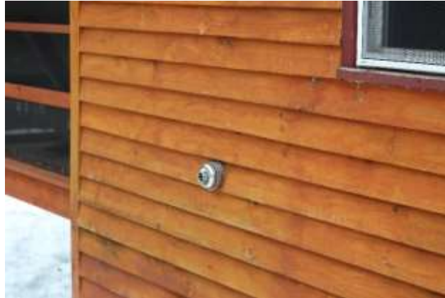
Figure 83 Propane Monitor Vent
