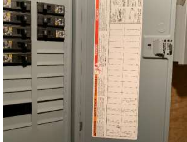
Figure 100 Labeling (wrong installation of cover)
