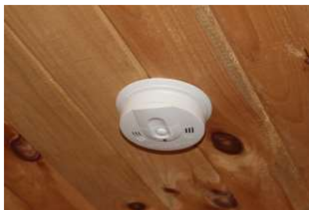
Figure 43 Combination Smoke/Co Alarm
