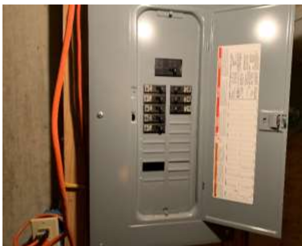
Figure 98 Missing Knockout
