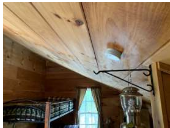
Figure 47 Smoke Alarm Location
