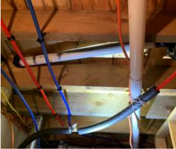
Figure 93 Plumbing Vent
