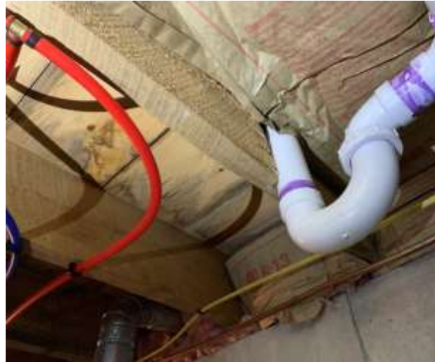
Figure 75 Cut/Broken Joist
