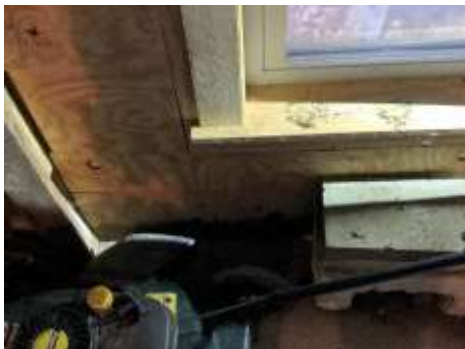
Figure 80 Active Water Intrusion
