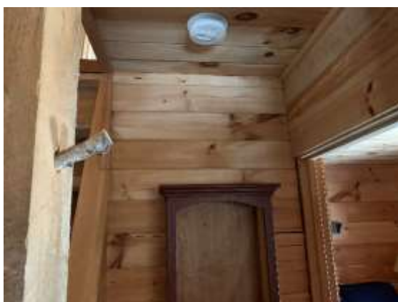
Figure 42 Combination Smoke/Co Alarm
