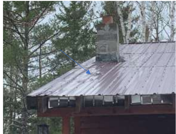
Figure 24 Damage to roof below chimney area
