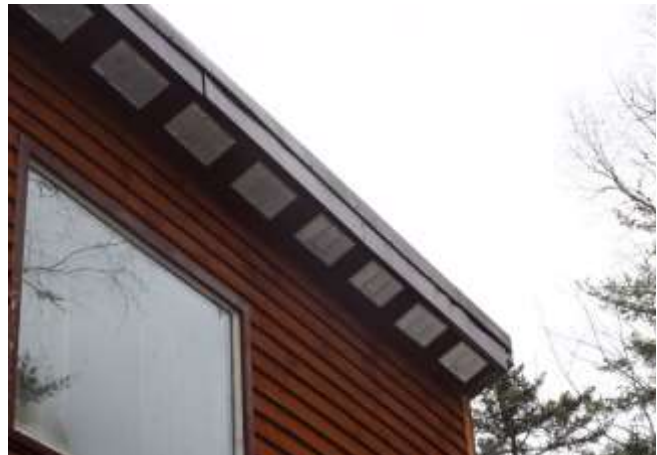
Figure 6 Vented Soffits
