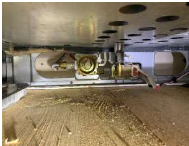
Figure 67 Lack of Anti-Tip Bracket
