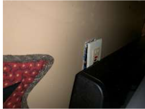
Figure 61 Loose Receptacle
