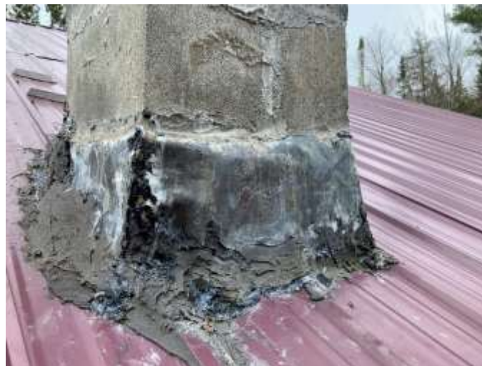
Figure 27 Improper flashing
