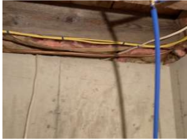
Figure 77 Poured Concrete
