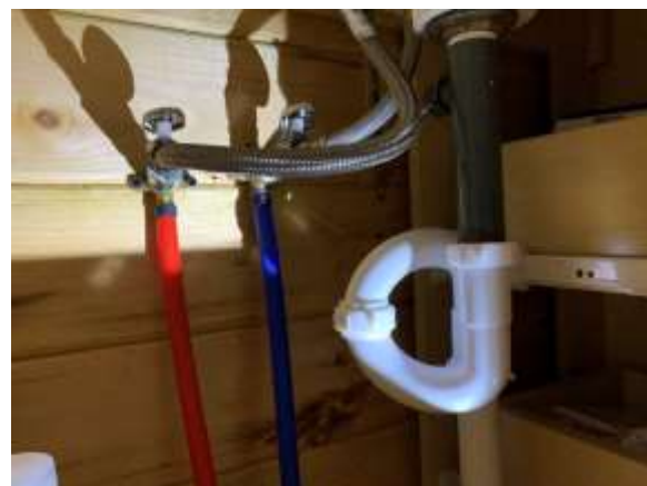
Figure 55 Improper "S" Trap
