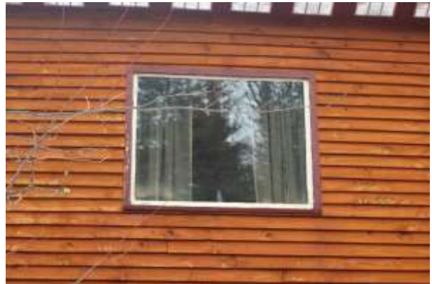
Figure 26 Missing Flashing at top of window
