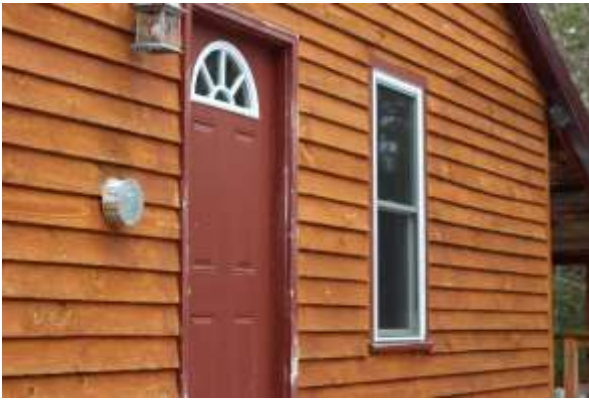
Figure 25 Missing Flashing at top of door
