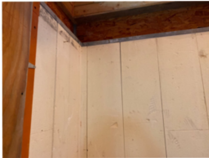
Foundation wall insulation
