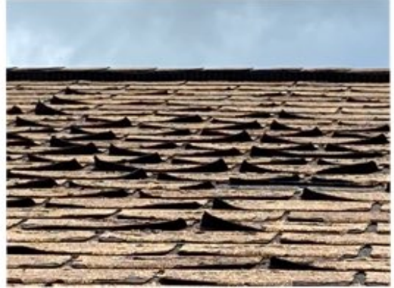
Curling asphalt roof shingles
