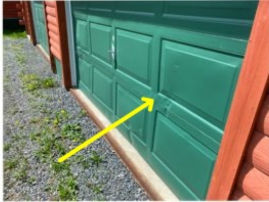
Mechanical damage to doors
