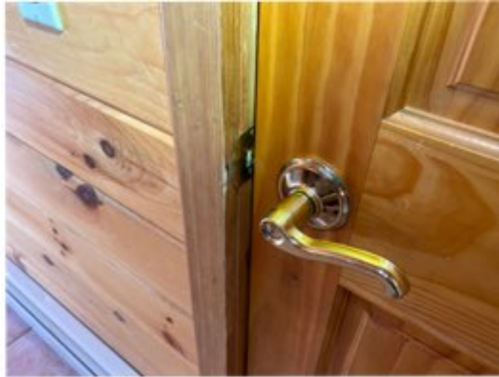
Basement door does not line up properly
