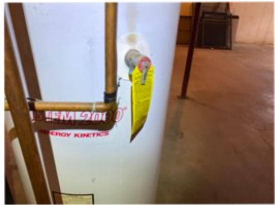
Missing Discharge pipe for TPR
