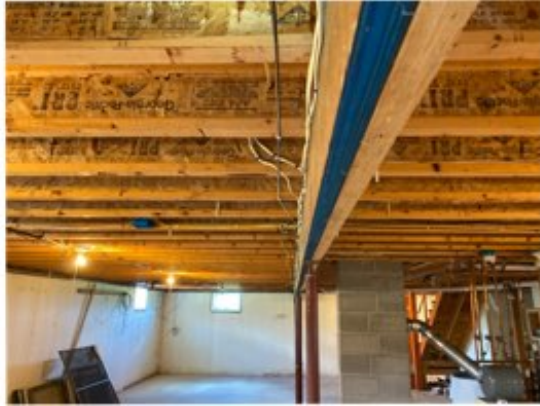
Manufactured floor joists
