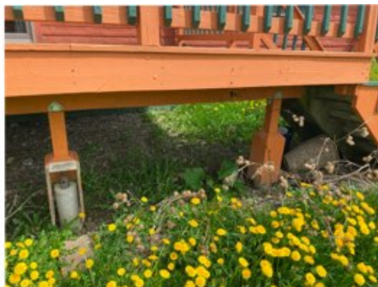
Inadequate supports
