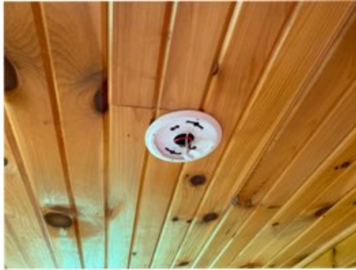
Missing Smoke Alarm
