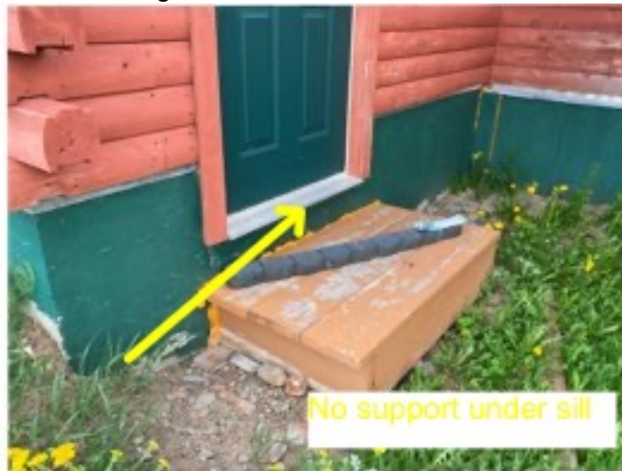
Inadequate support
