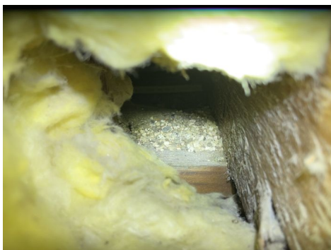
Possible vermiculite insulation under the batting
