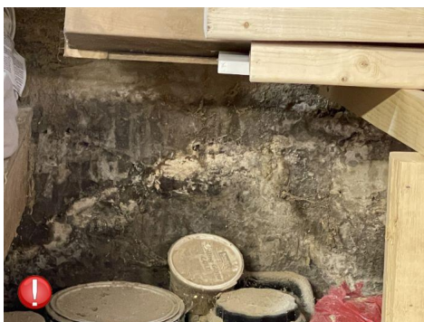
Efflorescence noted
