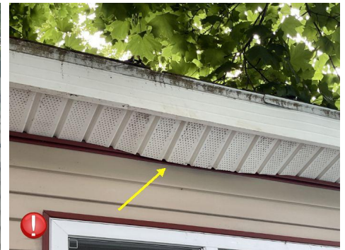
Loose materials at soffit
